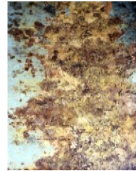
Fuel Tank Corrosion
