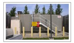
Core also supplies systems to store diesel fuel for critical emergency power. Our systems are readily adaptable for use in multi-generator and/or multi-tank control designs.
