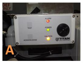
Photo A – When the Cube reaches a level of approximately 85% full, the red alarm light and the yellow caution light on the system display will be illuminated accompanied by an audible warning. This audible alarm is designed to notify the filler that the tank is nearly full.
