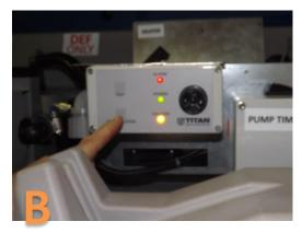
Photo B – To silence the alarm, press the acknowledge button once.
