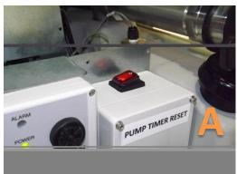
Photo A – Assure that the toggle switch is in the "ON" position.
