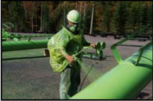
EPDM rubber coatings are very effective for protecting concrete pipe against salt water corrosion. They can tolerate higher temperatures, exposure to strong sun, and have 2.5 times higher solids than liquid Neoprene coatings.
