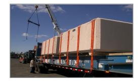
ConVault aboveground tanks are precast concrete units with a painted or architectural finish. The unloading equipment and procedures are critical to setting the tank safely and without damage to the tank.
